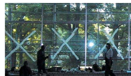
Installation of glass windows in first-floor multi-purpose space
