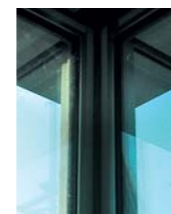
Connection of glass fin to reinforced-concrete slab
