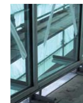
Glass fins used to stiffen facade assembly
