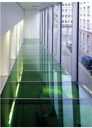
Glass ramp: green glass floor with view of ground 4 m below
