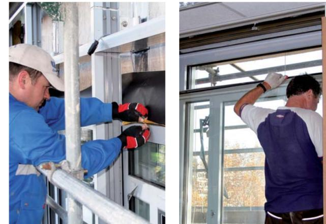
New window units are sealed (left) and old windows dismantled from inside building (right)
