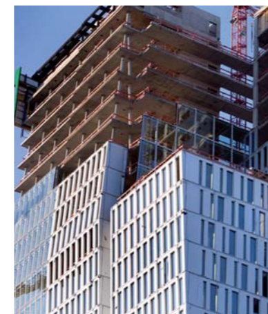
Office tower under construction and nearing completion ...
