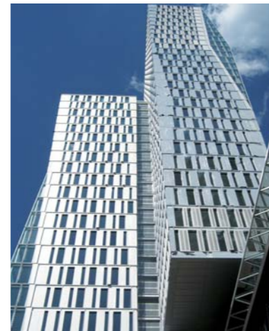
Eastern and western front of office tower with double-skin facade (left) and single-skin facade (right)
