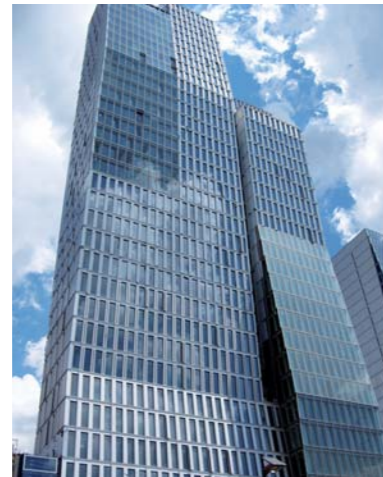
Eastern and western front of office tower with double-skin facade (left) and single-skin facade (right)
