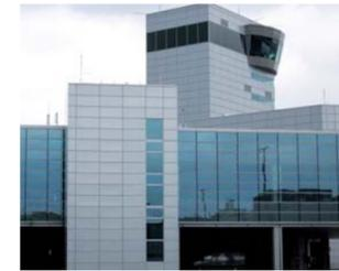
levels. Externally, these steel columns are faced with high-grade F90-fire-rated panels. The rhythm of the passageway exterior is interrupted by a staggered arrangement of ribbon windows. The rooftop plantrooms are clad in corrugated metal. The passageway component of the scheme was specially designed and built to cater for the possible future extension of individual facade areas. The fire-rated curtain walls are similarly adaptable to the evolving needs of a major airport.
