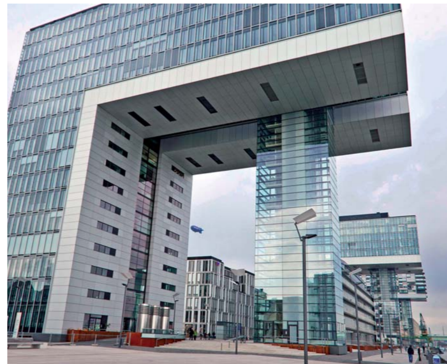
View through southern and middle crane houses towards Pandion Vista
